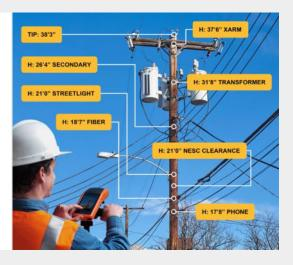
"Designed from the ground up to set the standard for measuring, locating and analysing utility poles for aerial fiber deployments, joint-use applications and construction of aerial outside plant."
